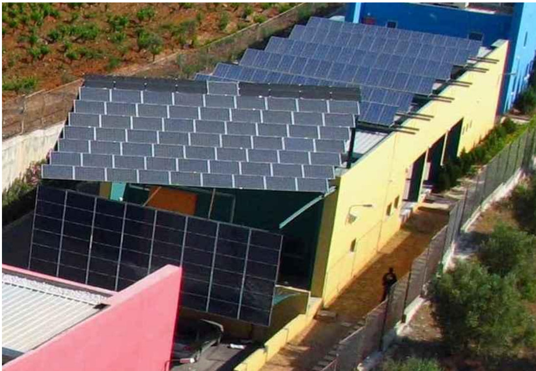
Figure 5: CRES, building of PVs and DER systems
